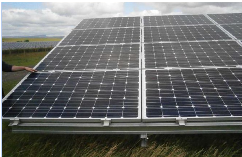
Figure 7-1 Typical Solar Panel Arrangement (showing expansion gaps)
